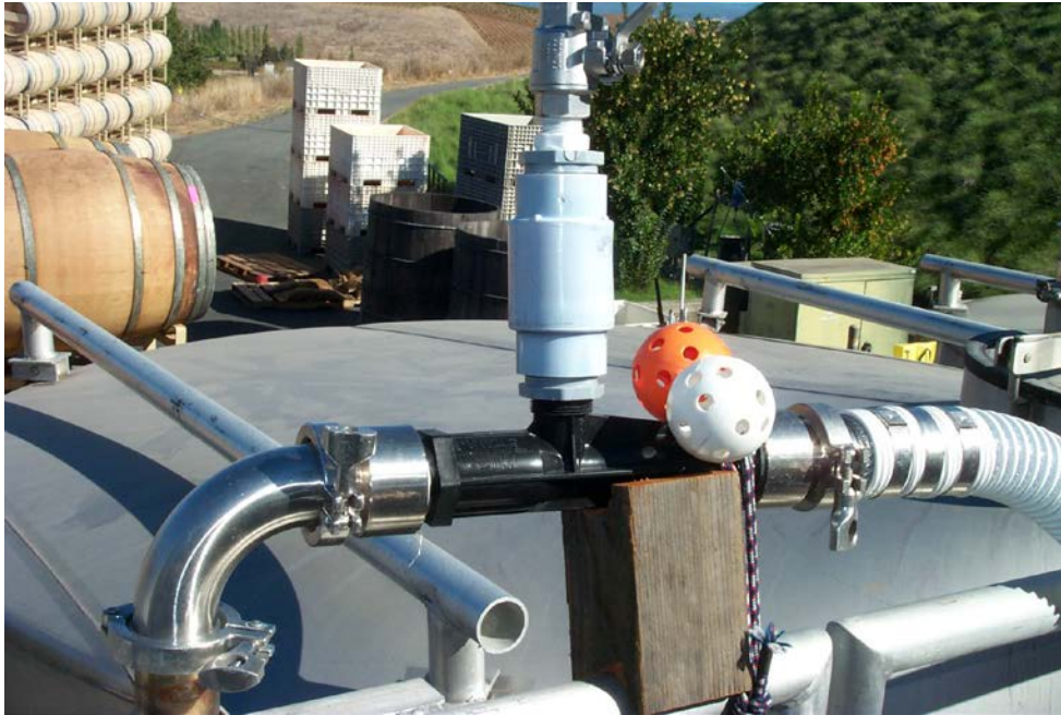
Mazzei Injector in place with adapters to Tri-Clover fittings and check valve.
