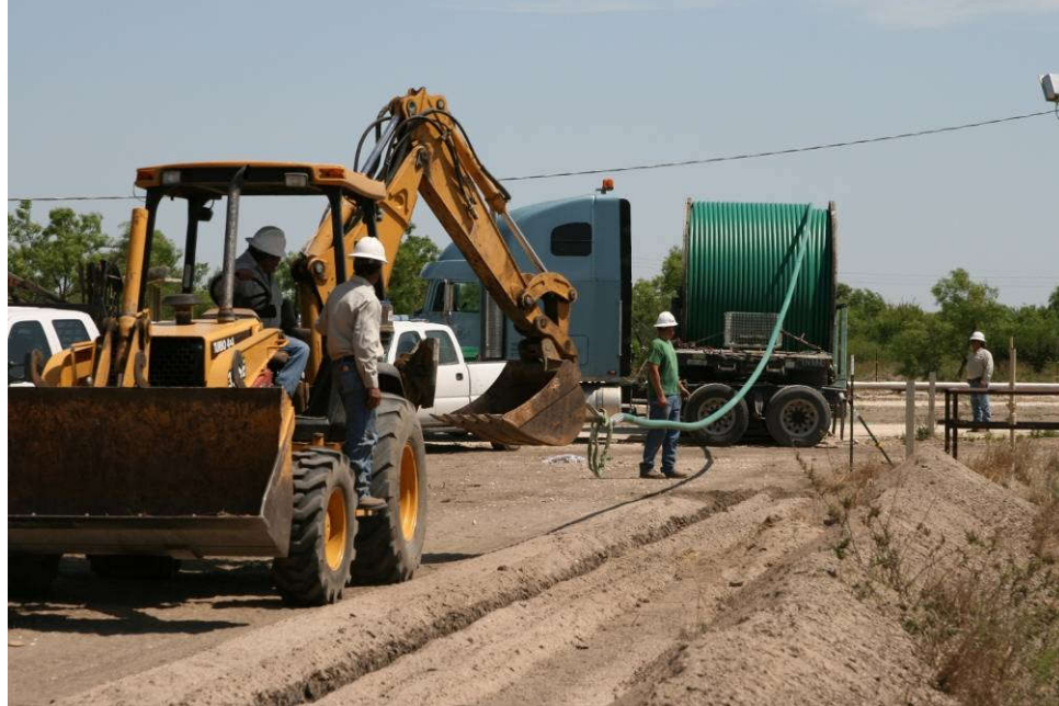
Figure 7-5 Spoolable Composite Pipe (SCP) - Unreeling Pipe for Placement in Pipeline Trench. (Photo used courtesy of Fiberspar LinePipe Canada Ltd)
