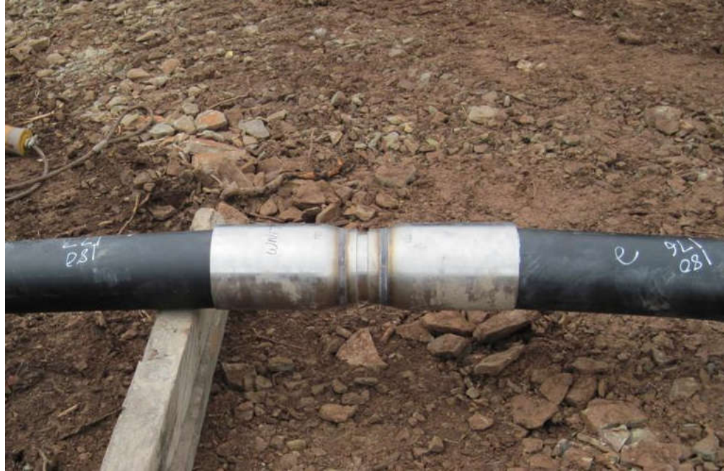
Figure 4-2 Spoolable Pipe Metallic Coupler Installation ( Photograph courtesy of FlexSteel Pipeline Technologies Ltd. )
