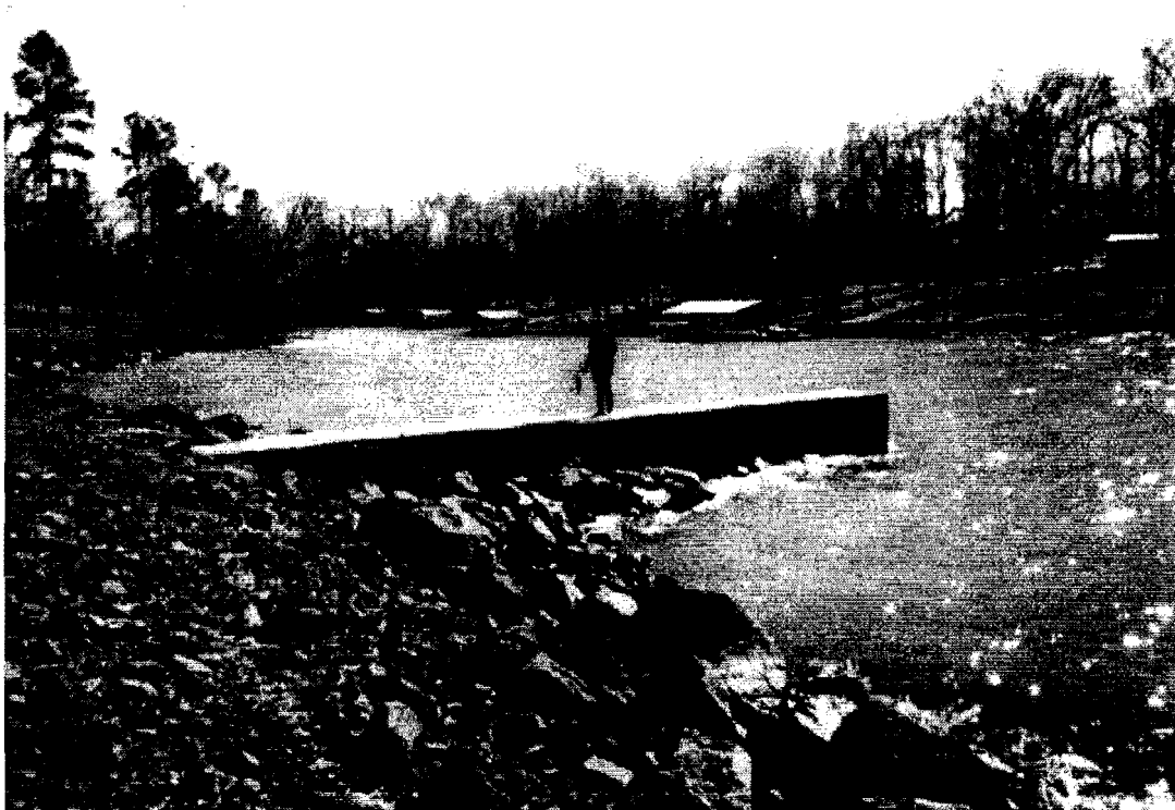
Figure 2.14: River Wing Dam Built Using Eco-Blocs (10)
