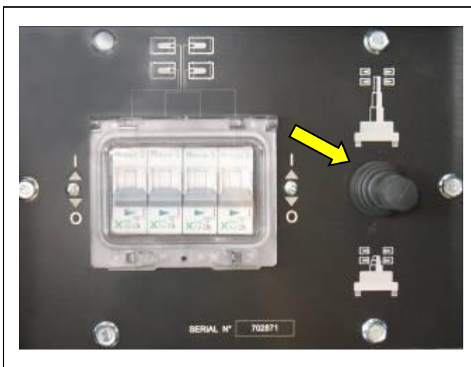
Figure 5.8 – Lowering the column
