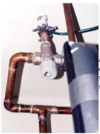
*Figure 6.* When water heaters are used for both space heating and domestic water, the domestic side must usually be mixed with cold water for safety's sake. A mechanical tempering value is a simple way to do this.
