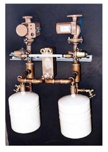
SuperStor's Voyager water heater works well in dual-purpose applications, for both drinking water and space heating. Voyager offers a built-in heat exchanger, but the author prefers to use an external unit, shown preassembled with expansion tanks and circulators in the photo (above left). The heat exchanger is fully insulated and is located between the tank and the red and blue heating loop manifold (above right).
