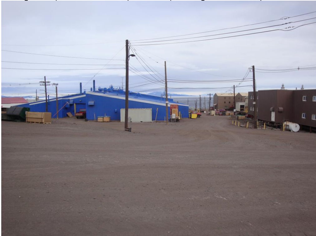
Building 155 from the NE with Building 211 (Lodging) on the right, looking SW along corridor to Derelict Junction
