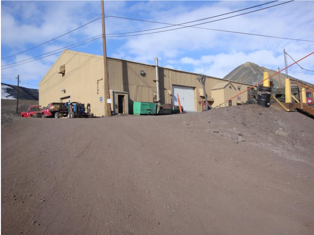
Building 136 (Trade Shop) from the northwest
