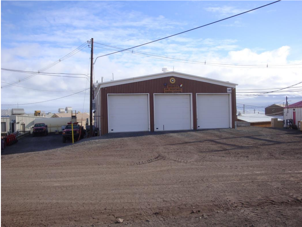
Building 182 (Fire House) from the northeast
