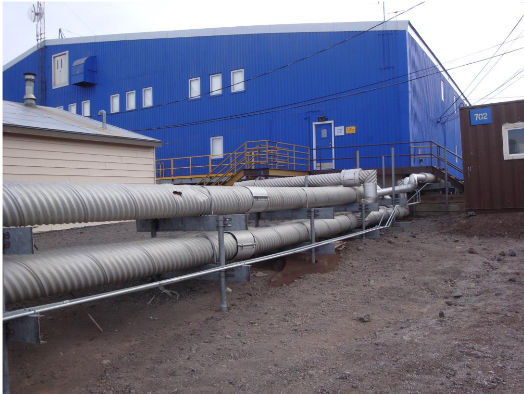
Utilidor looking north at the south corner of Building 155
