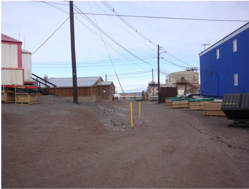
Looking SW with Buildings 142 (MAC Medical), 108 (Gallagher's), 189 (JSOC), and 155 in the background
