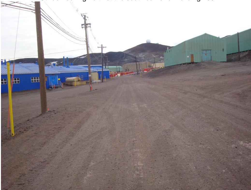
Looking NW at Building 155 and Building 120 (Food Warehouse)
