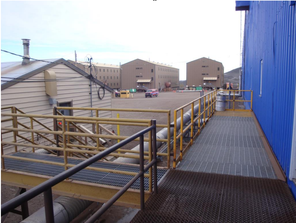
Looking west from south platform of Building 155 with Building 107 (Southern Exposure) and uppercase lodging
