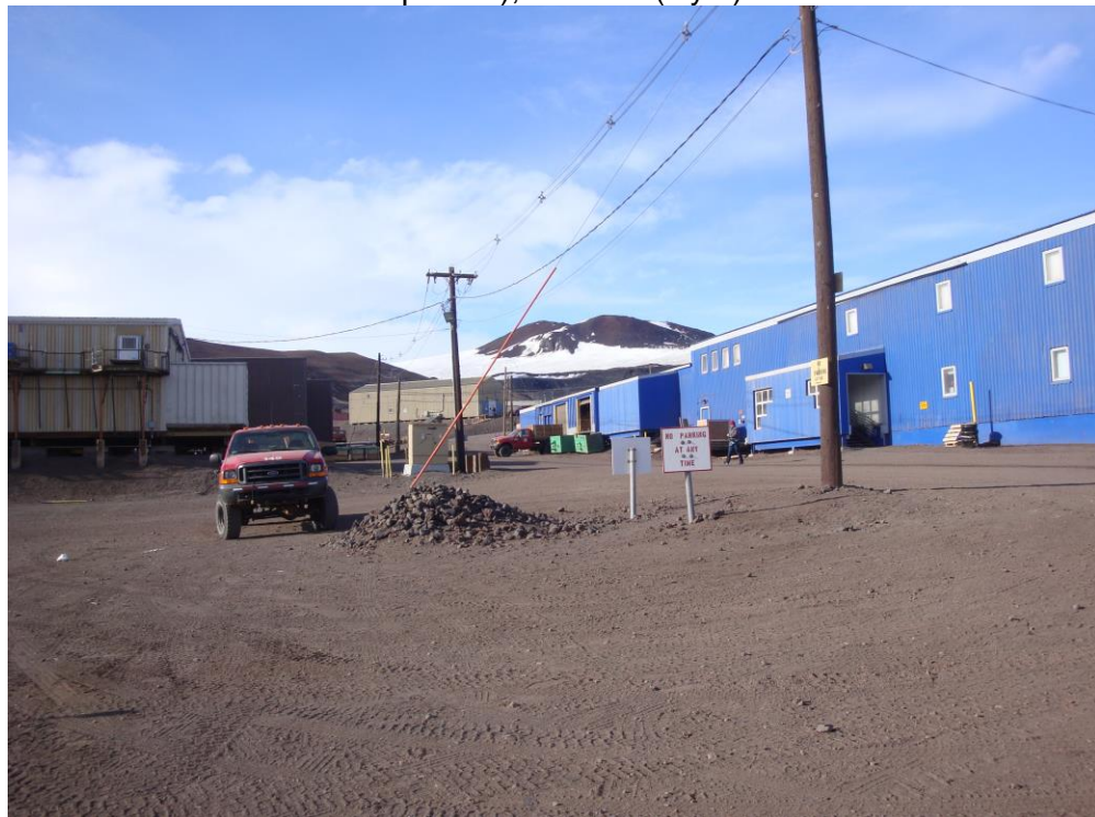
Derelict Junction looking NE with Building 164 (Frozen Food Warehouse) on the left and Building 155 on the right
