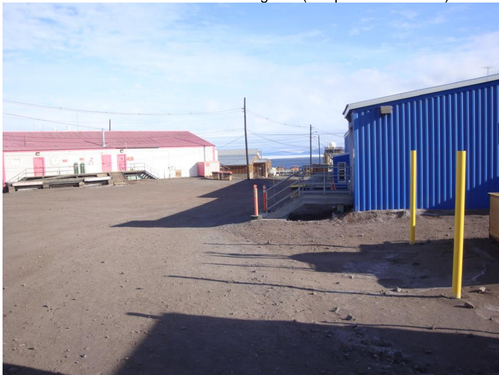
NE corner of Building 155 looking SW with Building 142 (MAC Medical) on the left
