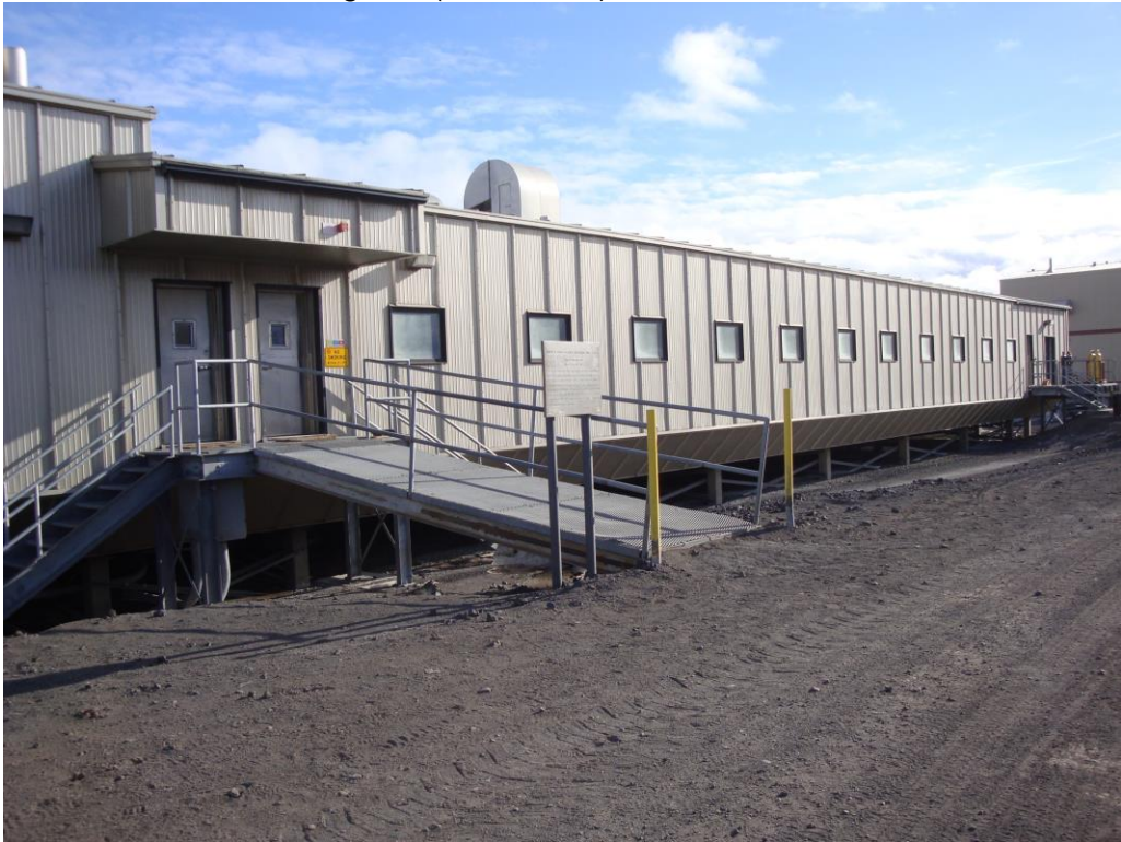
North face of Building 001 (Crary Lab) from the east
