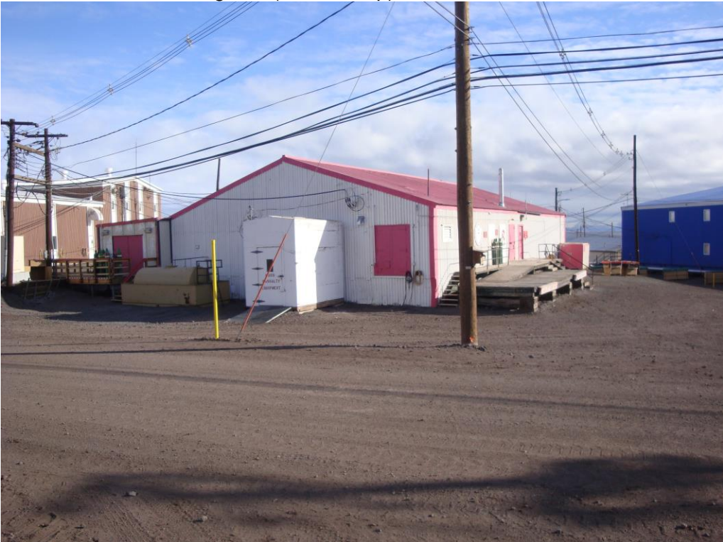
Building 142 (MAC Medical) from the east
