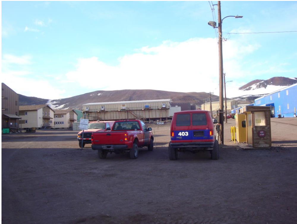
Derelict Junction looking NE with Buildings 206 (Lodging), 203 (Lodging), 164 (Frozen Food Warehouse), and 155 in the background
