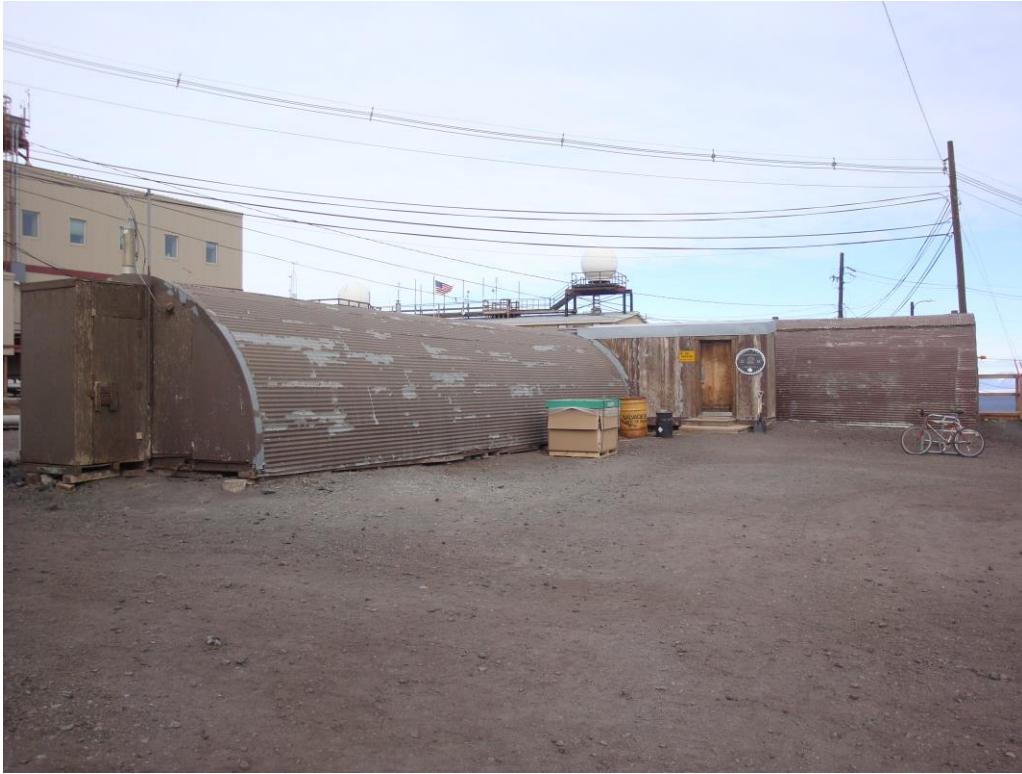
Building 076 (Coffee House) from the north
