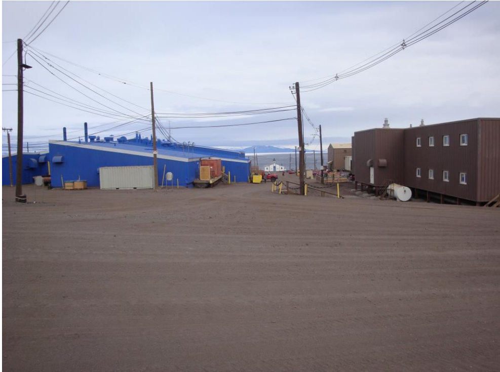
Building 155 from the NE with Building 211 (Lodging) on the right, looking SW along corridor to Derelict Junction and Building 007 (Chapel of the Snows)
