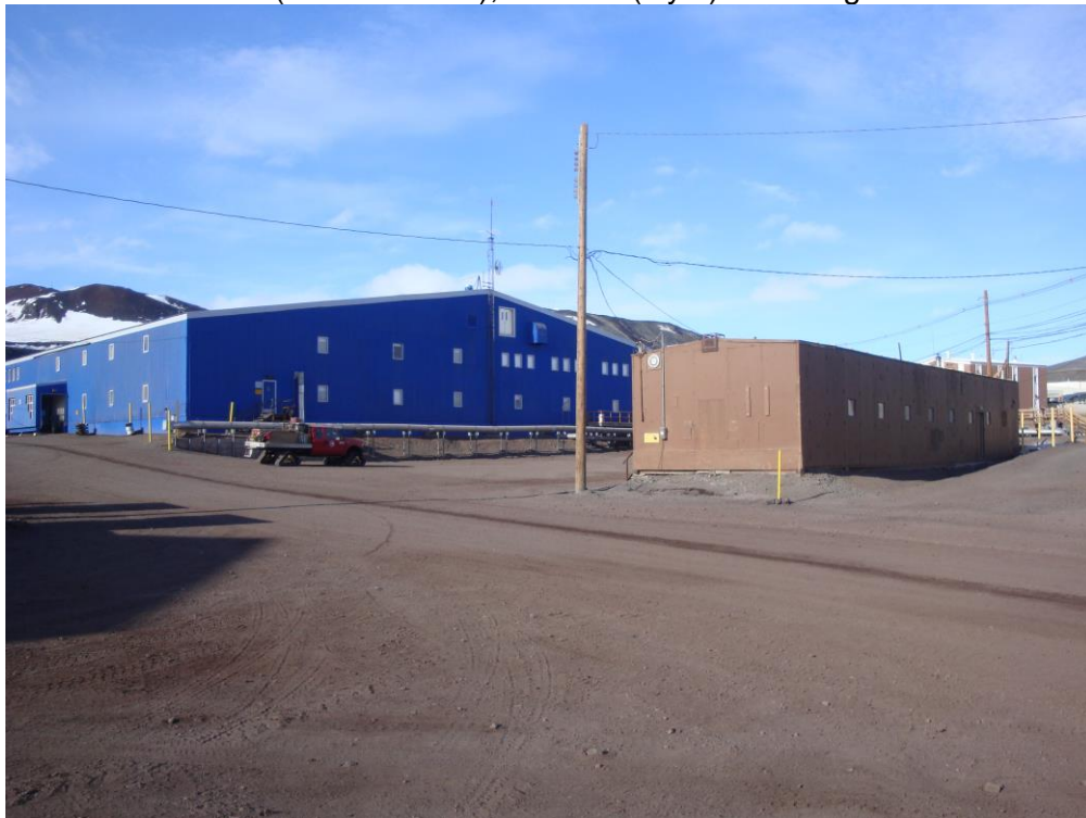
Buildings 155 and 078 (Gym) from the southwest
