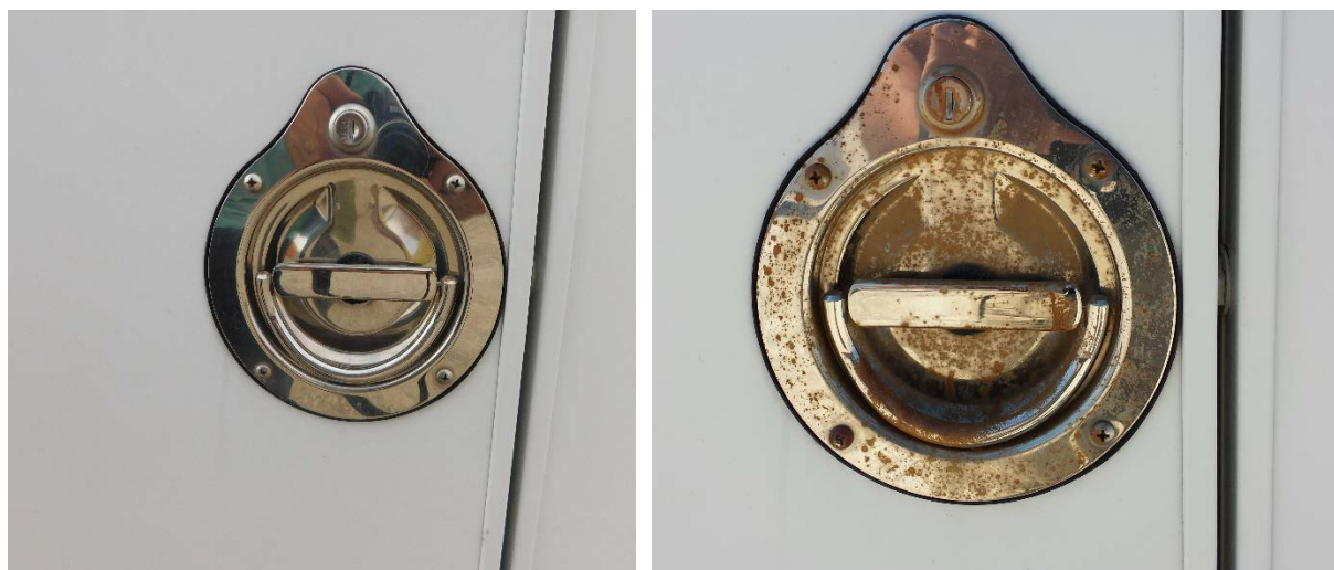
Figure 19b. Before exposure (left) and after one exposure (right). Notice the immediate corrosion.
