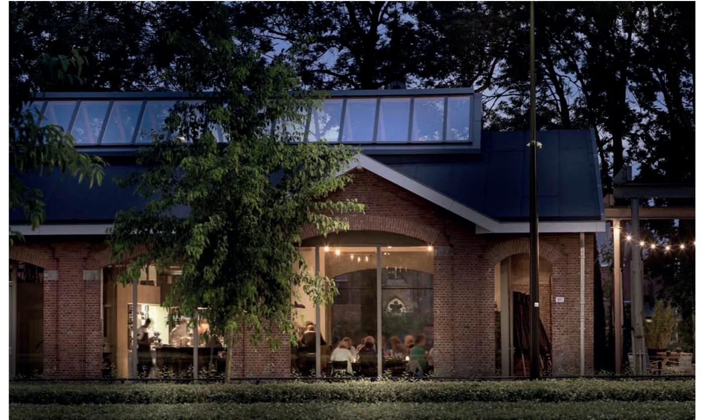
The Houtloods (transformation of old railway warehouse), Tilburg, the Netherlands. 124 modules.
