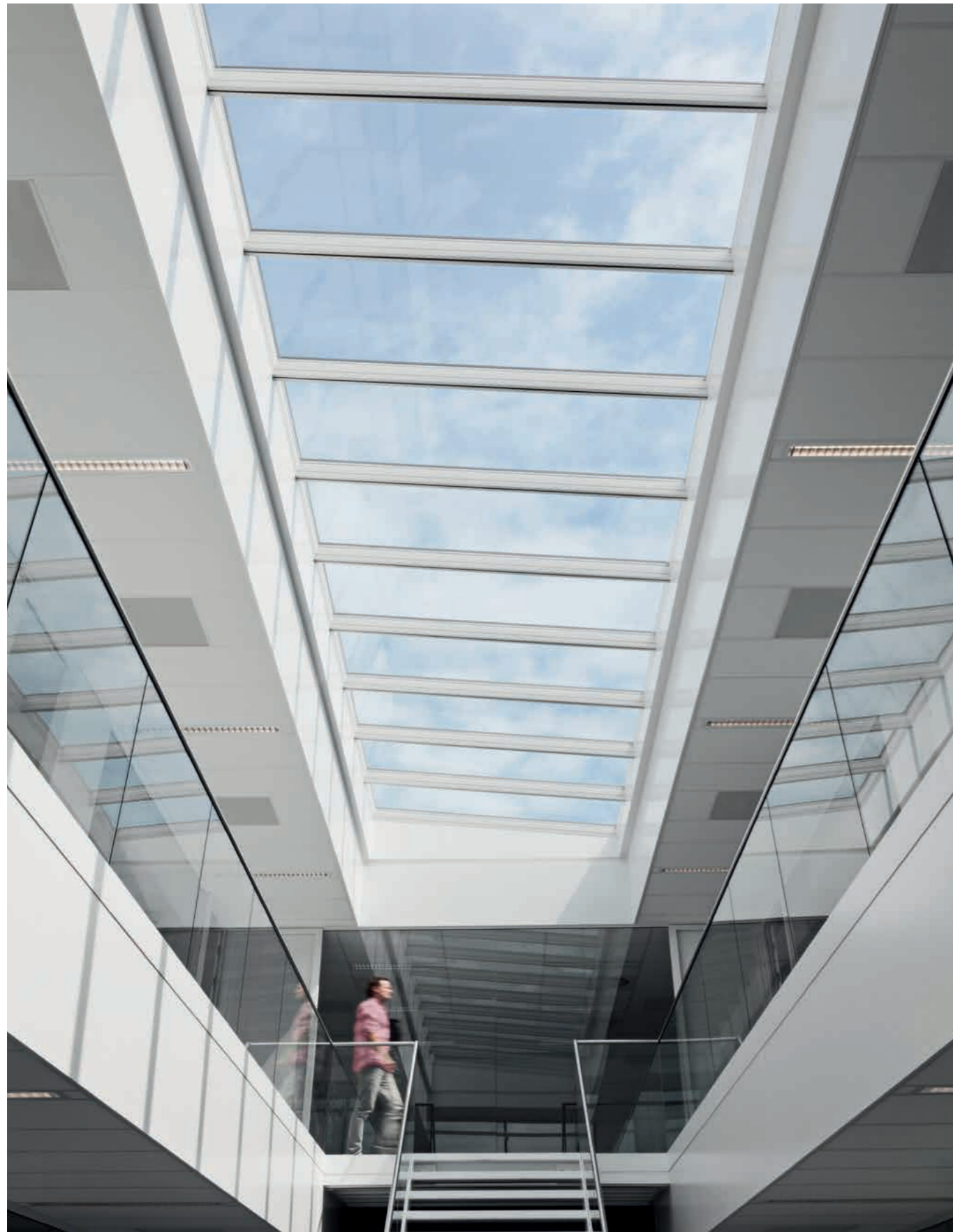
ASSA ABLOY office, Apeldoorn, the Netherlands. 12 modules.
