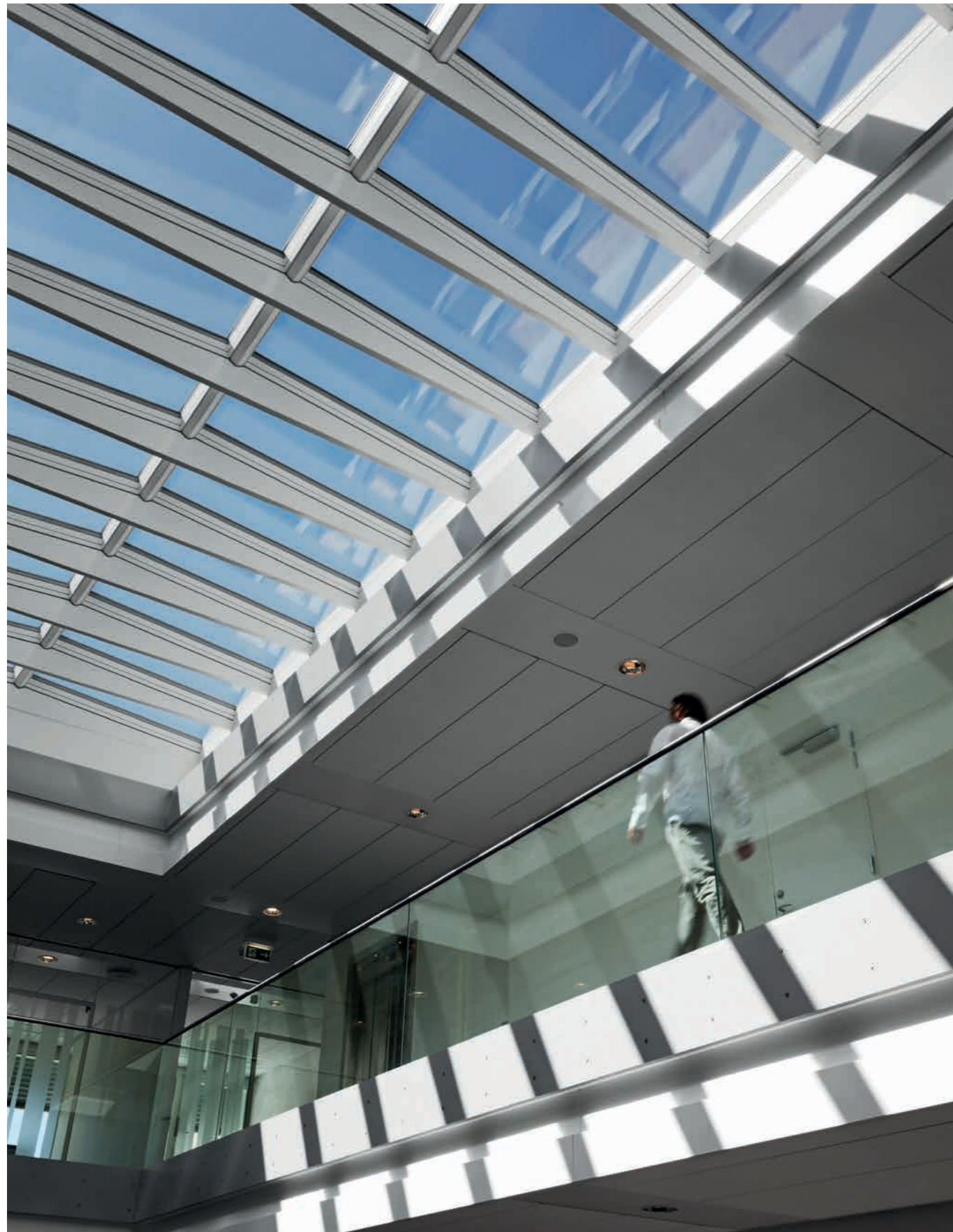
ATP, Vordingborg, Denmark. 26 modules.
