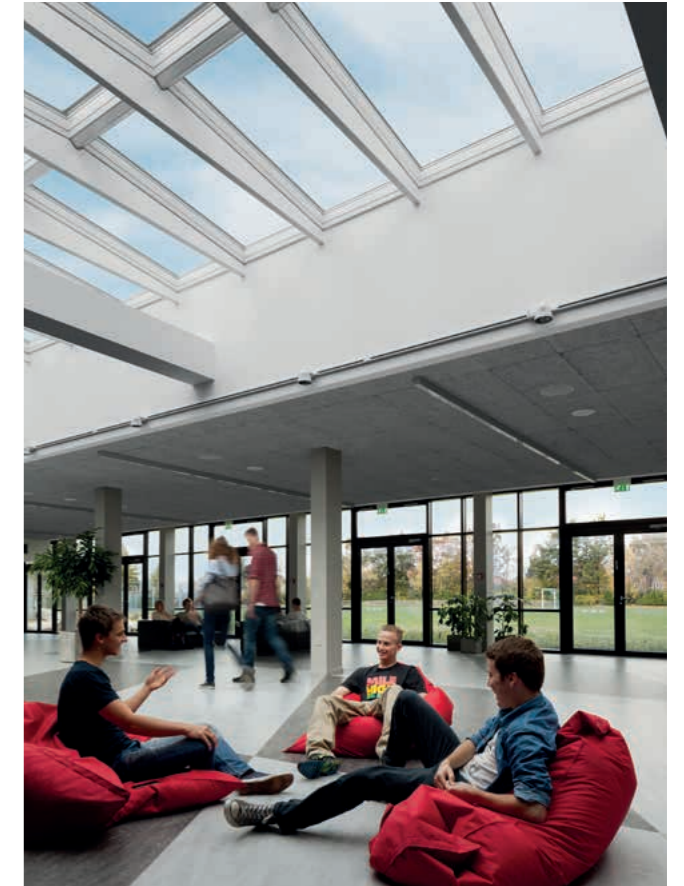
Roskilde Cathedral School, Roskilde, Denmark, 36 modules (assembly hall).
