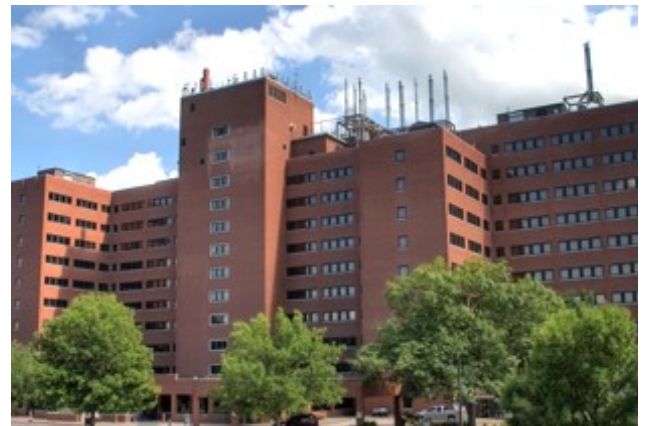
Iowa City Health Care System—Main Campus
