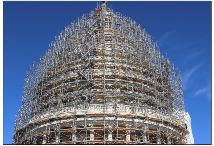
Scaffold-covered Capitol dome during renovation
