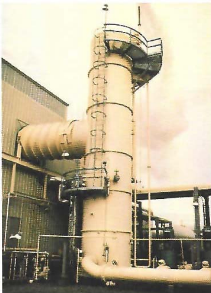
Direct contact geothermal condenser for 9 MW plant.
