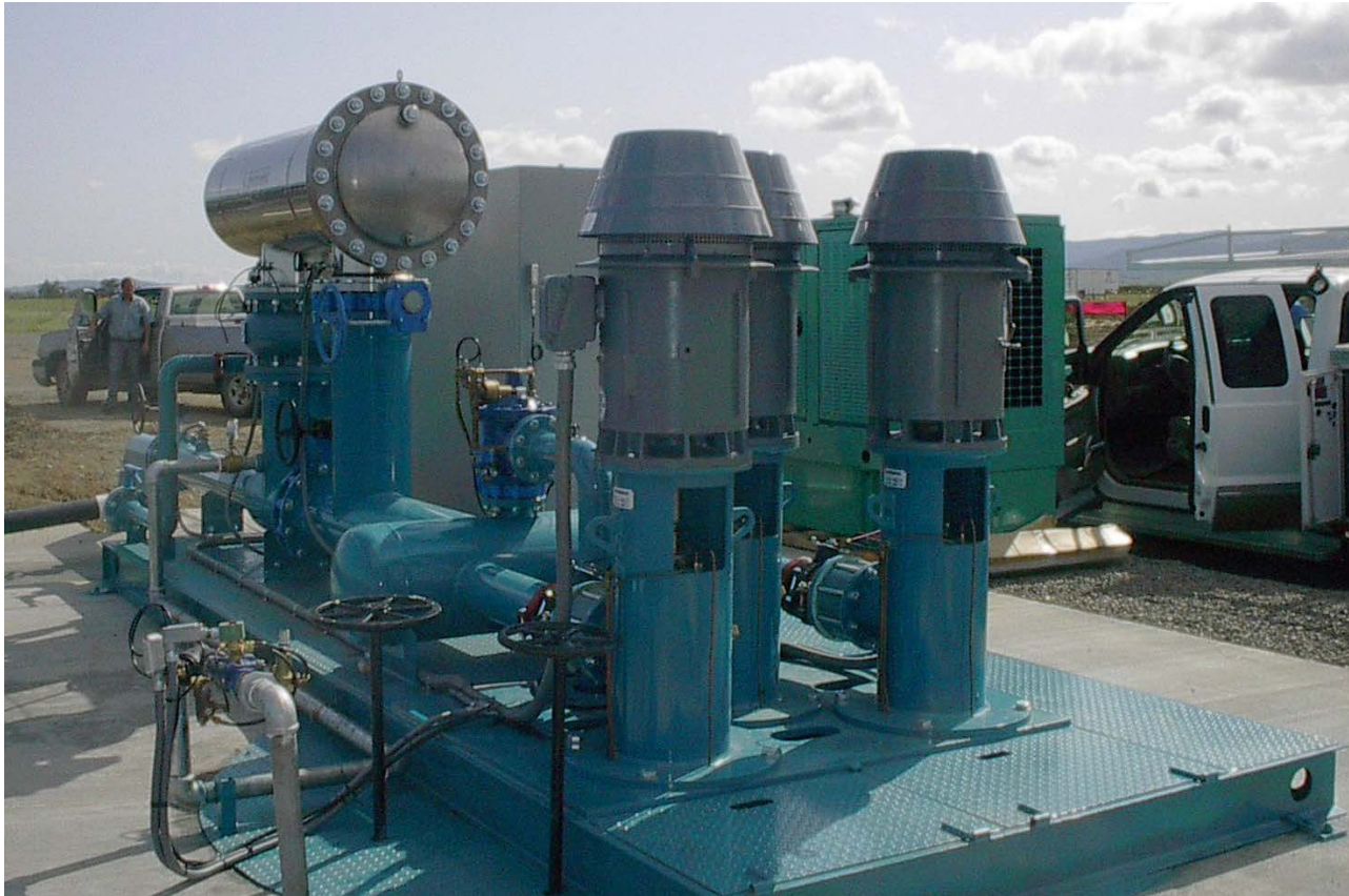
Nursery, Winters, California V-2000 200 micron 454 m 3 /hr (2,000 gpm) Recycled Runoff for Irrigation
