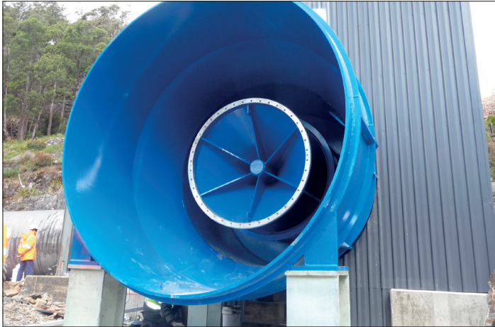
Picture 5: VAG KSSplus Howell-Bunger® Discharge Valve with pipe hood
