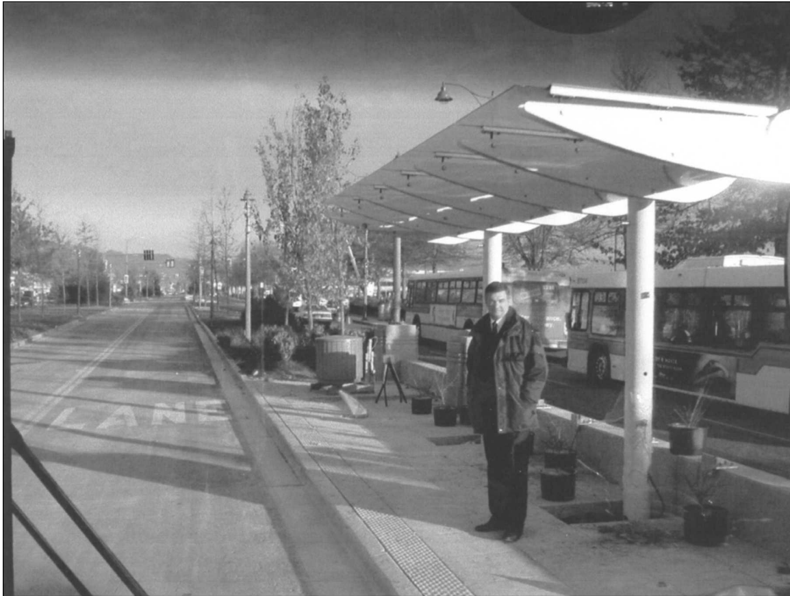
Figure 7: View of Busway Station – Richmond
