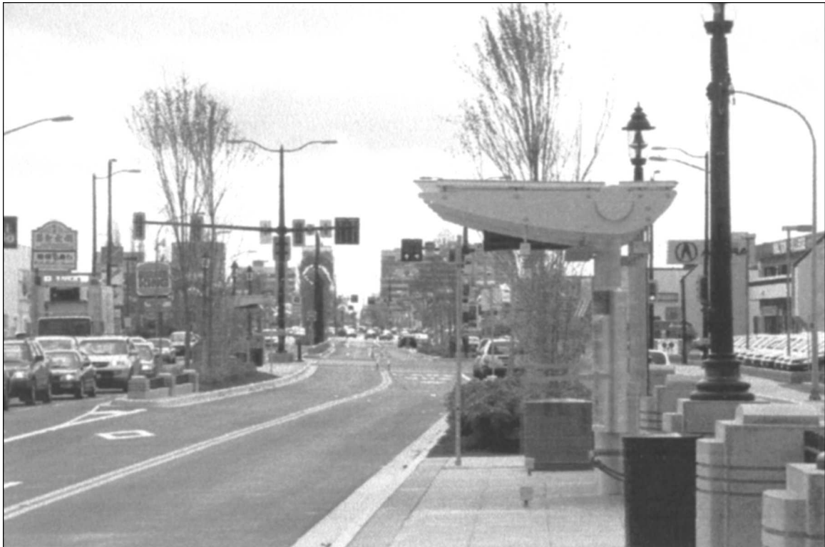
Figure 5: View of Median Busway – Richmond
