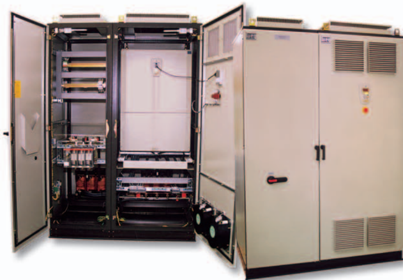
Inverter 361A, mounted in cabinet, controlling a 150kW-Motor for conveyor
