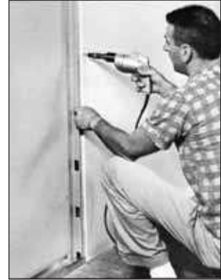
Kal-Kore boards are screwed to steel studs or nailed or screwed to wood studs to form a base.
