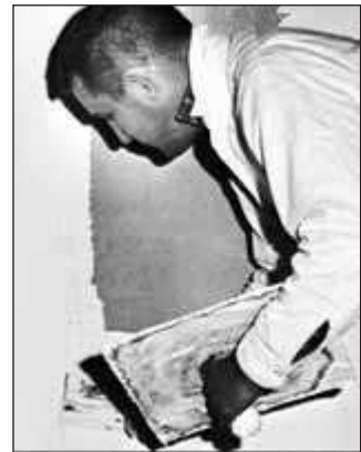
Kal-Kote is applied in 2 coats, a base and a finish, to form a hard-surfaced, 1/8" total thickness.
