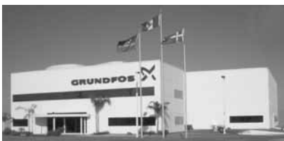
GMX - Monterrey, Mexico
