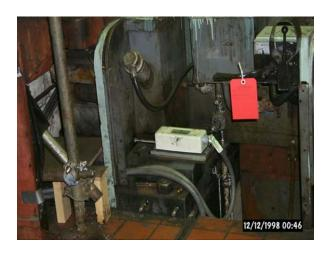
Differential Expansion measurements are an important parameter receiving much attention during turbine startup and warming. This parameter measures how the turbine rotor expands in relation to the turbine shell, or casing. A new differential expansion system using Eddy Probes can be retro-fitted to any existing system. An Eddy Probe is more reliable and robust than OEM supplied induction coil systems.
