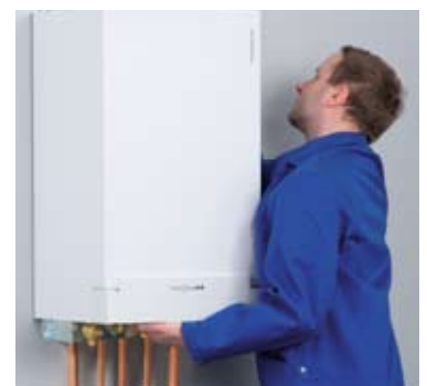
2. Mounting the boiler
