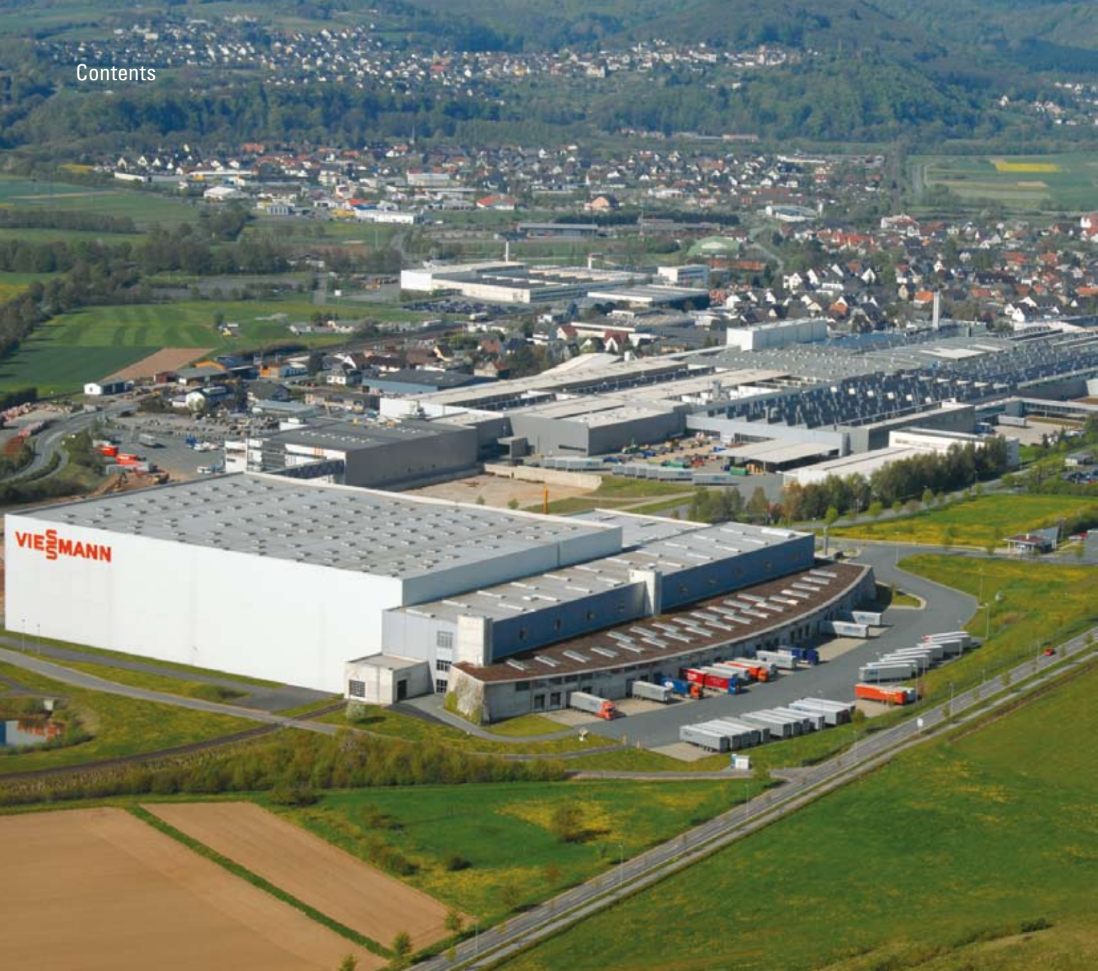
Viessmann Headquarters, Allendorf (Eder), Germany
