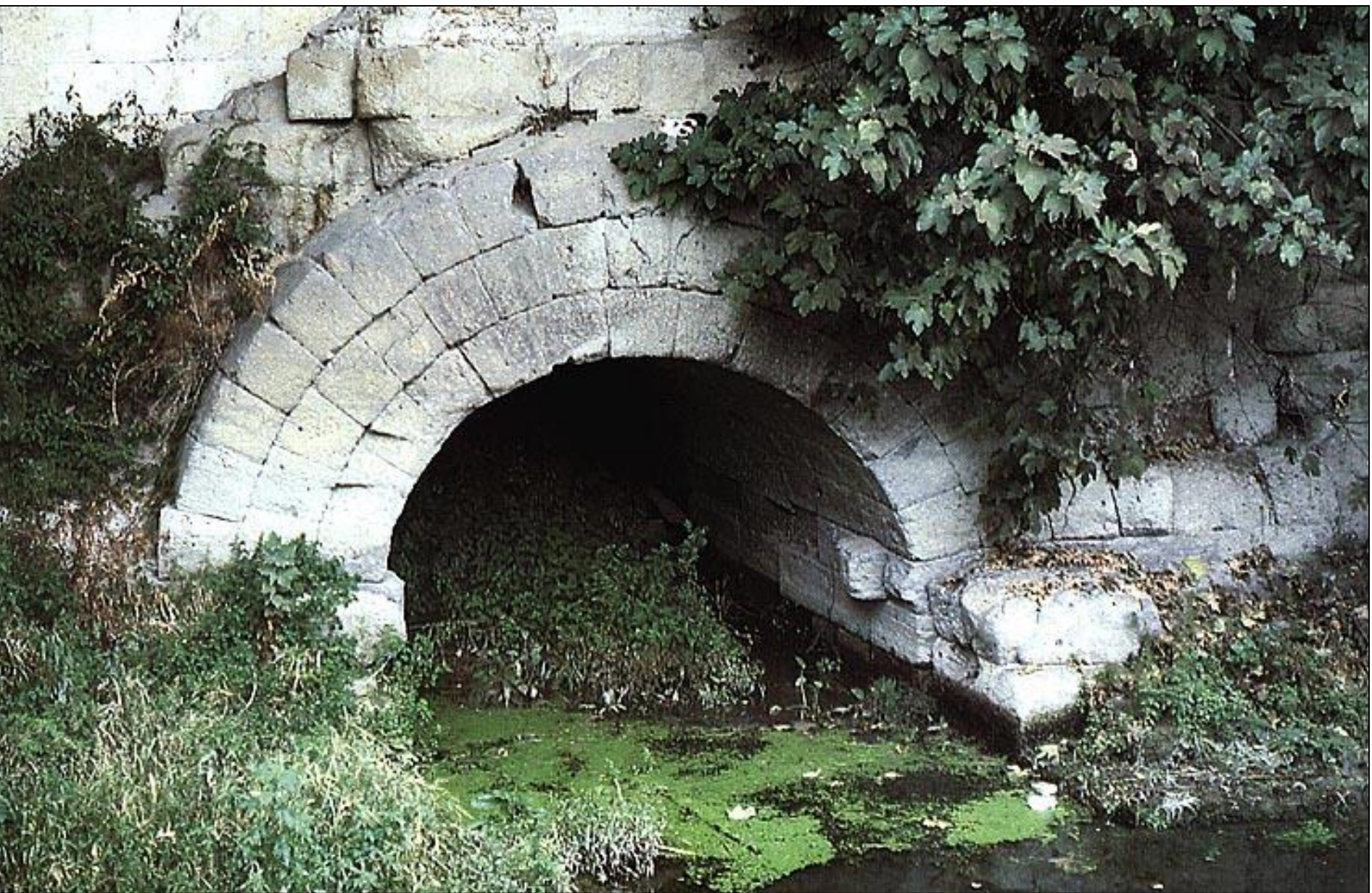
Cloaca maxima -- "the big sewer" draining Forum
