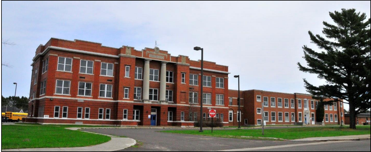
Figure 11: Acquired Ontonagon Elementary School Property
