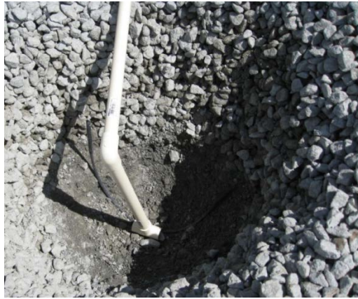
Figure 4: Temperature Probes Being Installed
