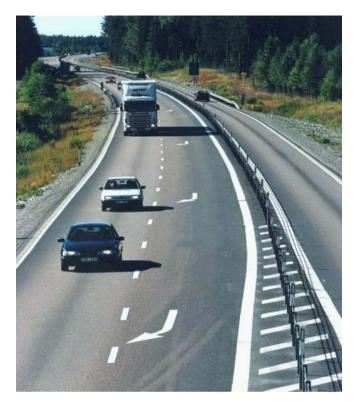
Fig. 3. A redesigned rural road in Sweden with 2+1 lanes and mid-barrier, resulting in a reduction of fatalities by 80–90%.
