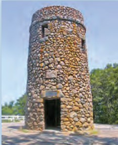
SCARGO HILL TOWER
