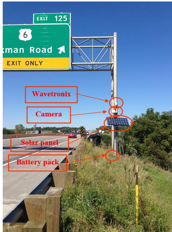
Figure 2. Example of Wavetronix detector and camera setup
