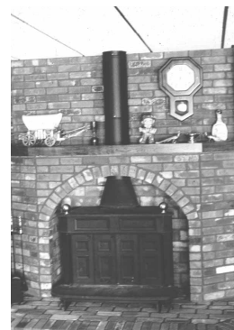
Figure 11. Wood stove as a local heating system
