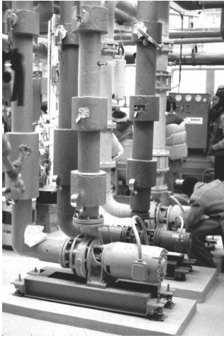
Figure 35. Centrifugal pumps.
