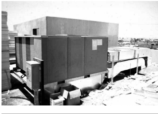
Figure 60. An integrated package, single-zone air-conditioning system.
