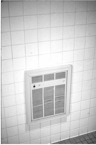
Figure 17. Built-in electric resistance heater.
