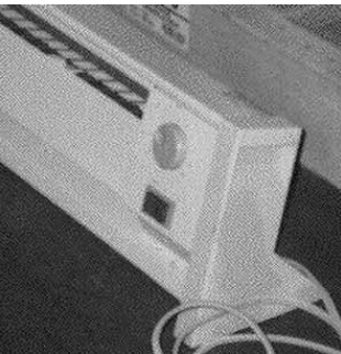
Figure 18. Electric baseboard radiator.
