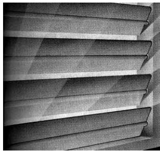
Figure 39. Air flow control dampers.
