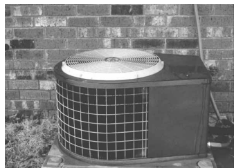
Figures 58. and 59. Exterior and interior (without cover) units of a split-system.
