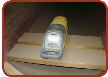
Figure 3: A common pipe laser in use
