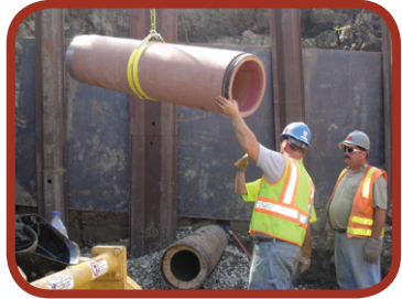
Figure 1: Lowering VCP Jacking pipe into the pit
