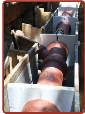
Figure 20: EPS foam blocks used in a full encasement installation.
