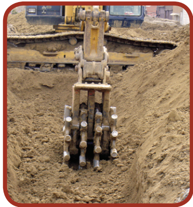
Figure 28: Close-up shot of a sheep's foot roller
