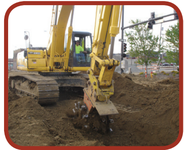
Figure 27: Hoe mounted sheepfoot roller compacting final backfill
