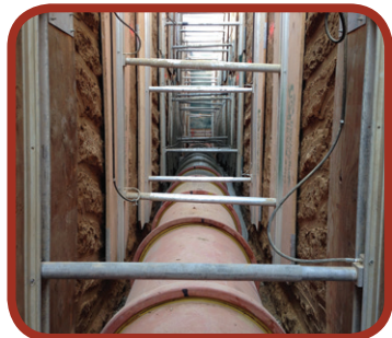
Figure 6: Trench sheeting and spreader bars
