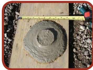
Figure 16: Measuring the spread diameter to determine flowability prior to placement
