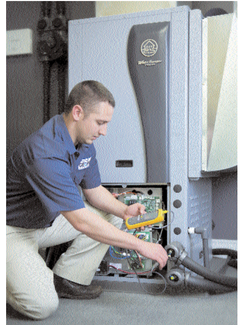
Provided by WaterFurnace International, Inc. By Scott Niesen
