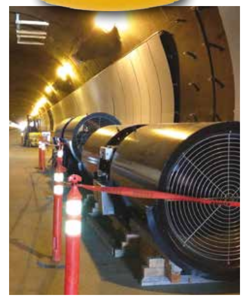
Jet fans to move airflow through tunnels.
