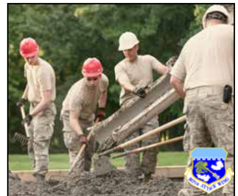
107th Civil Engineer Squadron Airmen pour concrete to create a ramp at the West Virginia School for the Blind and Deaf in Romney, W. Va., June 21, 2018.
