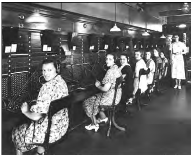
Bell Telephone Company operators at their switchboards in Owen Sound, which many rural companies connected through, 1937.
