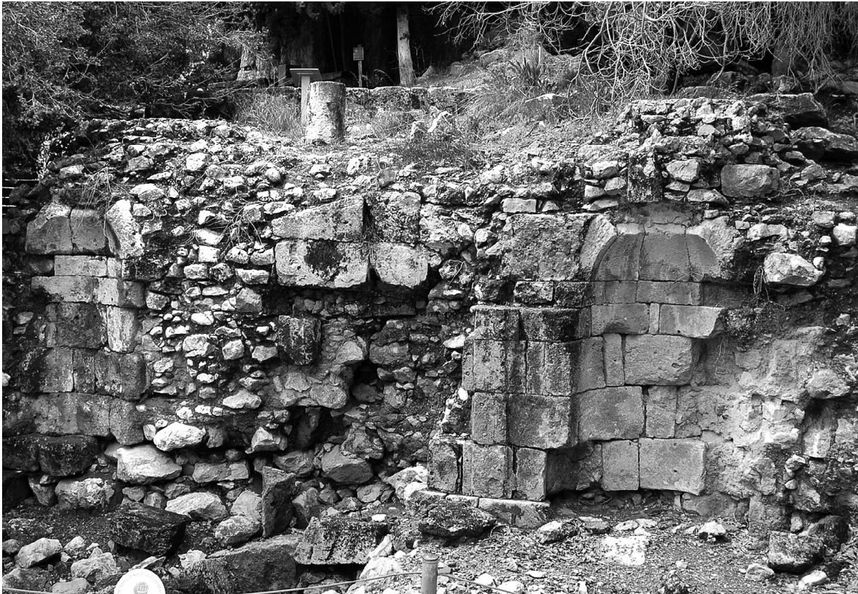
Fig. 5. The Paneion's opus quadratum wall along the cliff edge in front of the cave (photo author)
