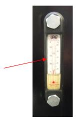
Fig. 15 – Hydraulic Fluid Sight Gauge.
