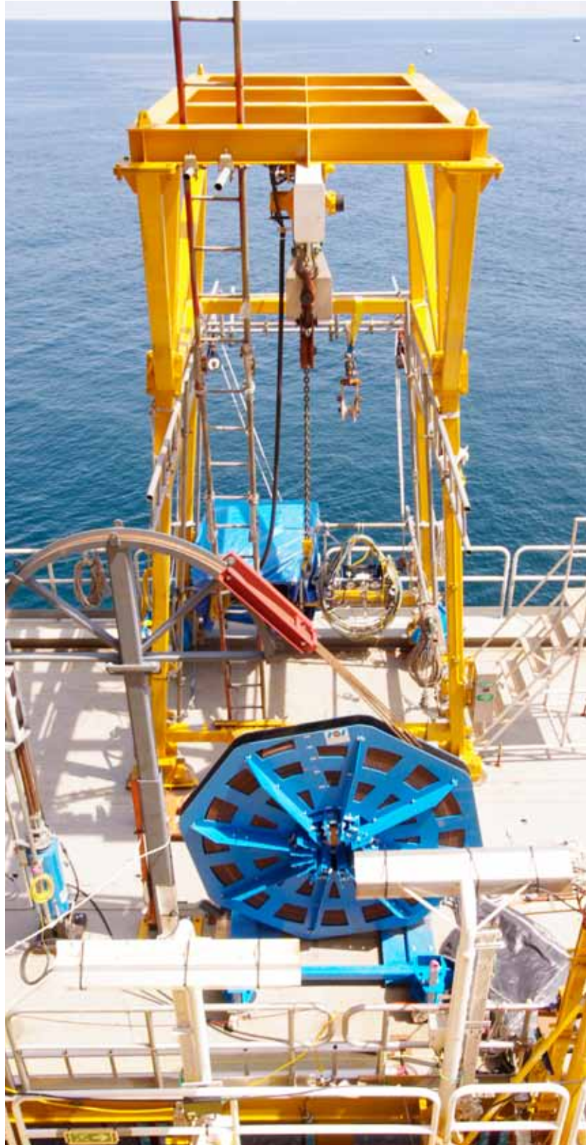
Risers and umbilical cables were lifted from a depth greater than 100 m onto a floating production storage and off-loading unit. The coilers for the operation were custom-made for the project. USAN Deepwater Development Project - Nigeria (2011)
