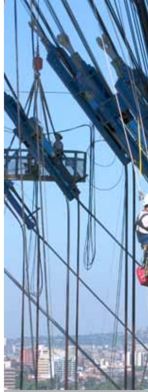
The roof structure of Warsaw's new stadium features a stunning central spire, two tension rings and 144 radial cables. The cable-net roof was lifted by 144 strand lifting jacks. Narod Stadium, Warsaw - Poland (2010-2011)
