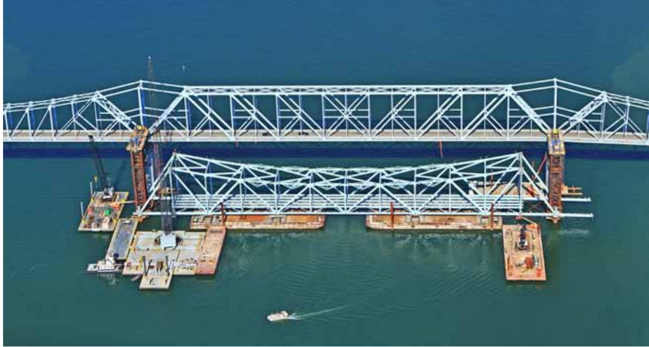
A complete 740 m-long bridge was slid laterally following an earlier operation to lift the two middle spans from pontoons. Milton-Madison Bridge, linking Indiana and Kentucky - USA (2012 and 2014)
