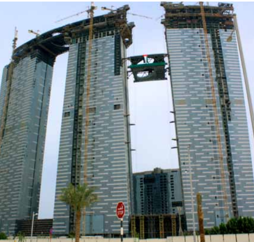
Building the world's highest 'sky bridge' involved lifting 750 t segments by 230 m. Gate District Towers, Abu Dhabi - UAE (2011)
