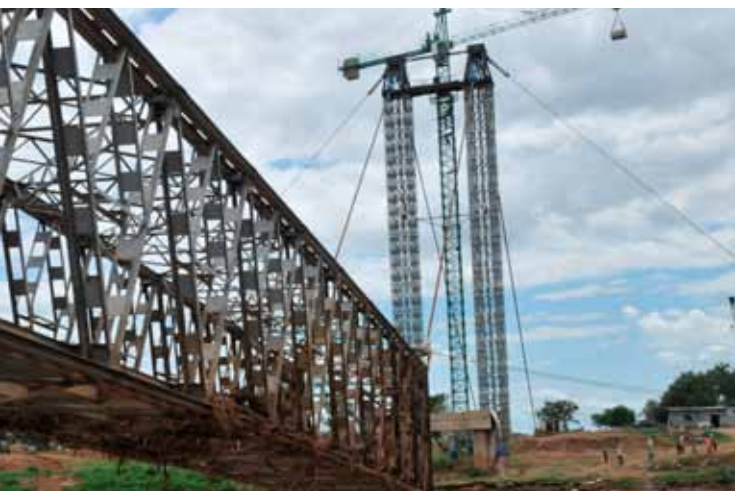
VSL was brought in to recover a 128 m-long steel bridge that had fallen into the river. The 550 t bridge was then launched 36 m into position. Omo Bridge - Ethiopia (2013)
