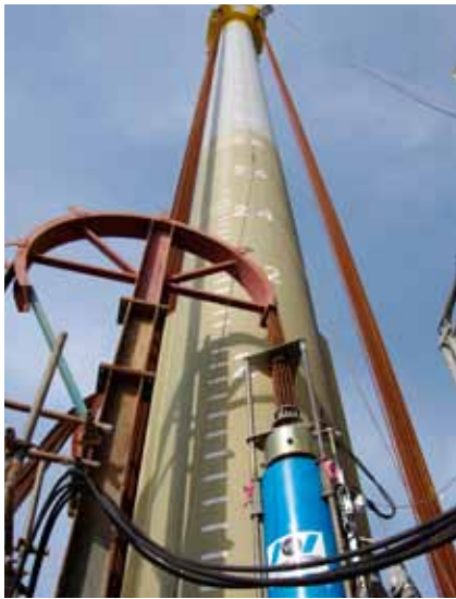
Offshore installation of a self-elevating leg barge required VSL to lift a 2,300 t hull and lower four support legs, each weighing 145 t. Sanaga Leg Barge - Cameroon (2001-2012)
