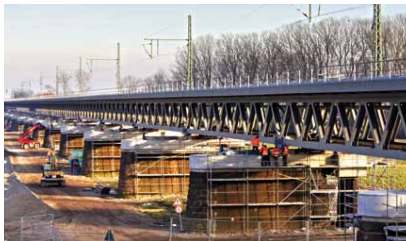
Launching and lateral sliding operations were carried out for a 606 m-long replacement railway bridge. Rheinvorland Bridge, Worms - Germany (2010 - 2012)
