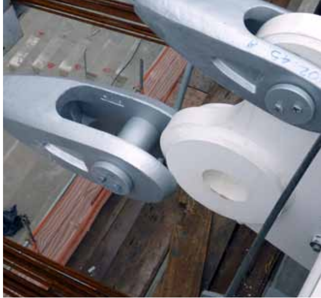
The last pin: one of the largest cable-net roofs in the world was raised into place using 60 lifting points. Maracanã Stadium, Rio de Janeiro - Brazil (2012-2013)
