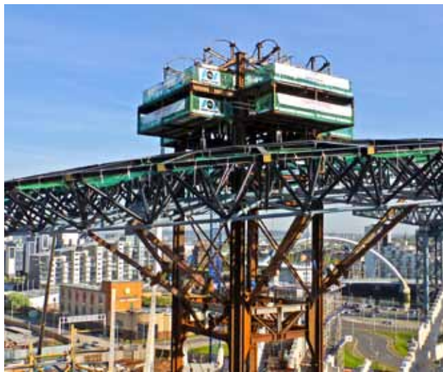
VSL carried out a complex operation to lift a 340 t steel roof, transfer the load onto the permanent bearings and install a lighting ring. SSE Hydro Arena, Glasgow - Scotland (2012-2013)
