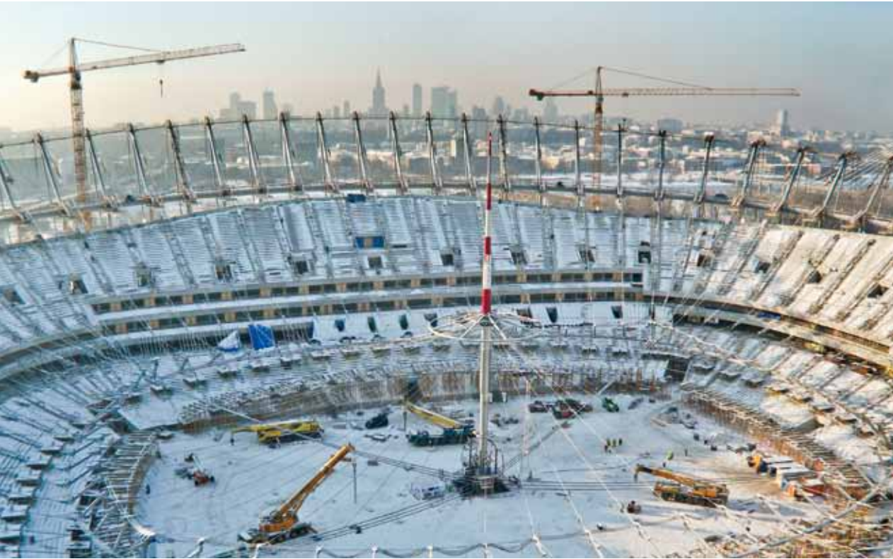
The roof structure of Warsaw's new stadium features a stunning central spire, two tension rings and 144 radial cables. The cable-net roof was lifted by 144 strand lifting jacks. Narod Stadium, Warsaw - Poland (2010-2011)
