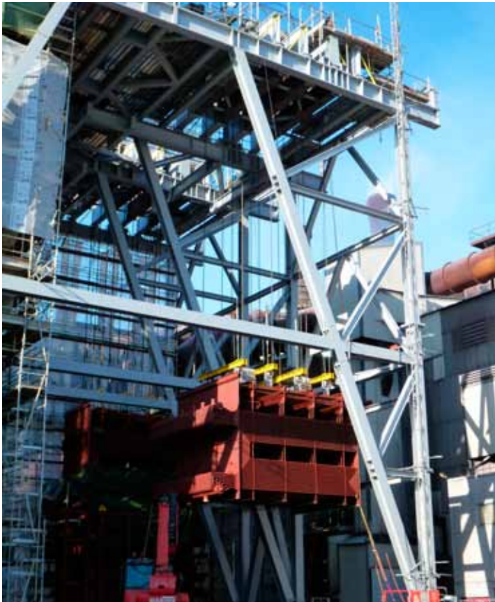
Four Aalborg boilers were lifted at the energy recovery plant of one of the most energy-efficient ferrosilicon producers. Finnfjord energy recovery plant, Finnsnes - Norway (2011 and 2012)
