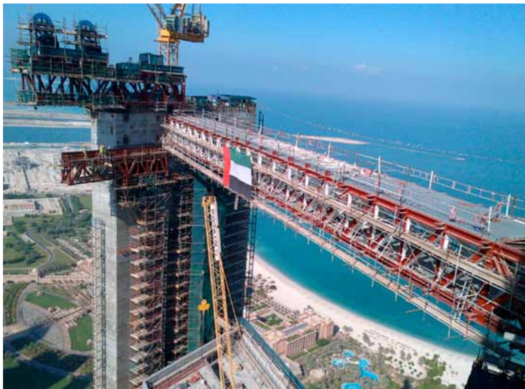
With a lifting distance of 335 m VSL Heavy Lifting broke a new record when it raised three roof trusses on top of the ADNOC's new headquarters building. The trusses were then slid into their final positions. ADNOC Building, Abu Dhabi - UAE (2013)
