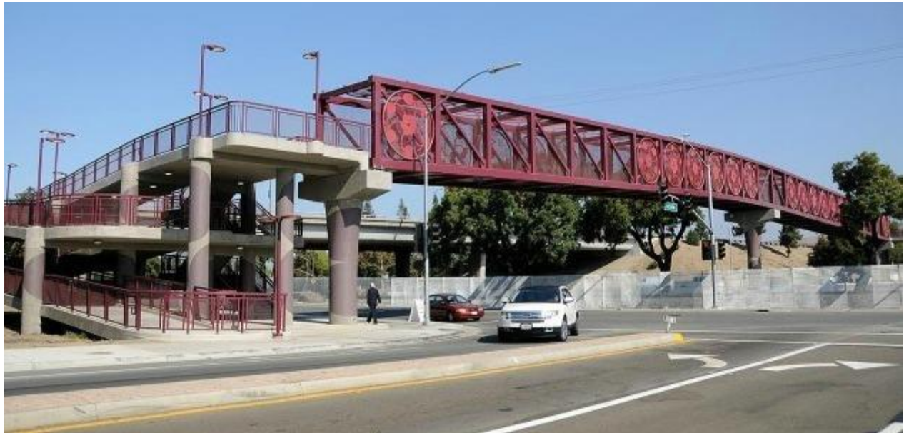
Blossom Hill Pedestrian Overpass, San Jose
