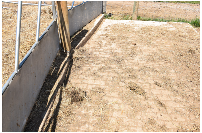
Figure 5. When using concrete feed pads, it is helpful for cattle traffic if the concrete is grooved to prevent slipping. Also notice the raised pad inside the hay feeder. At a height of 6 inches, this pad allows moisture to move away from the feeder but also reduces any mud or manure from seeping under the feed panels. (Photo credit: Matt Webb).
