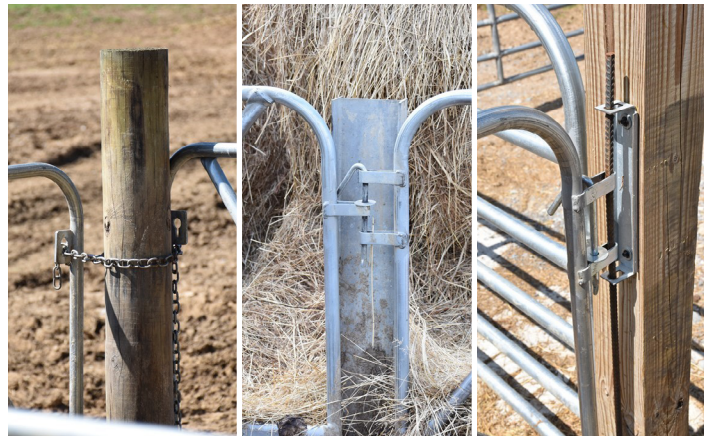
Figure 6. Different brackets used to install feed panels. The hinged and pin brackets when supported by a post were more rigid than attaching with a chain. (Photo credit: Matt Webb).
