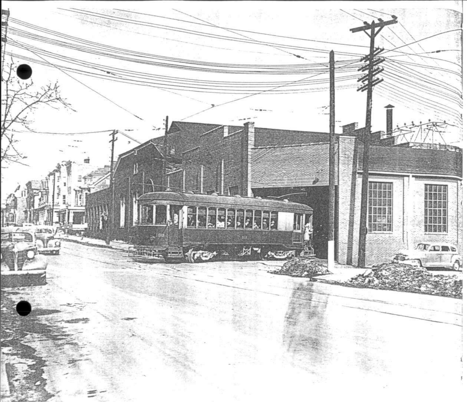
The big brick Hagerstown carhouse started life in 1898 as the Hagerstown Railway's power plant. After loss of the original carhouse in 1917, it was rebuilt to service the trolleys. The structure stood at Summit Avenue and Lee Street. — W. E. JOHNS
