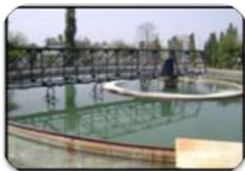
Clarifluculator (Sedimentation)
