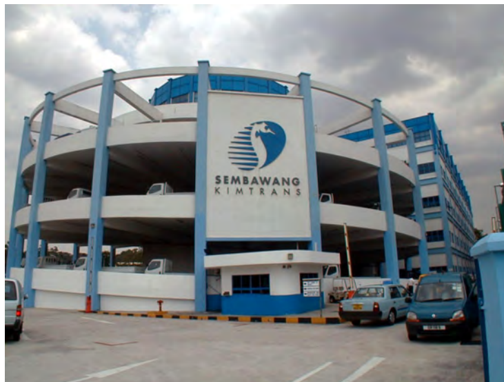
Figure 16.5: Multi-story warehouse with no automation but accessibility provided by a spiral truck ramp.
