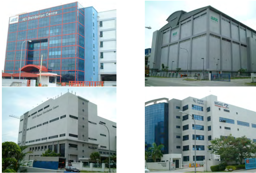
Figure 16.4: Multi-story warehouses are common in Singapore, Hong Kong, and Japan where land is expensive.
