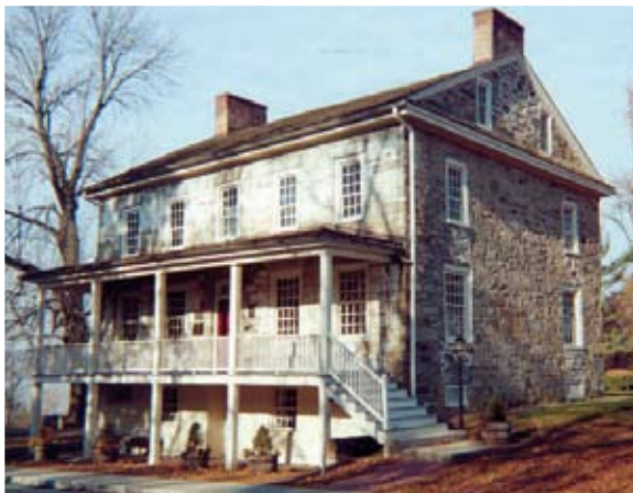
Examples of historic buildings along the route. Top to bottom: Aquia Church, Virginia; John News Ordinary, Virginia; Roger's Tavern, Maryland.
