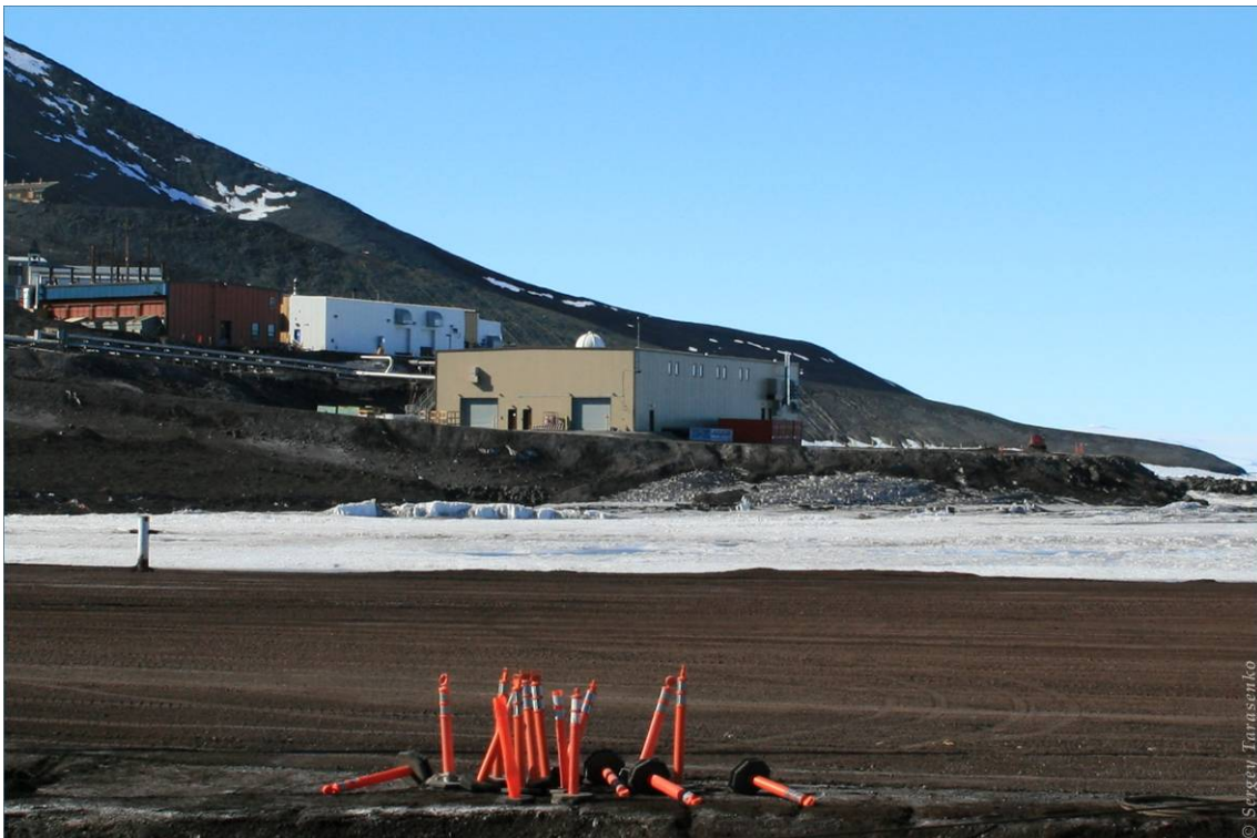
Figure 3 – Wastewater treatment plant building at McMurdo station (2008)
