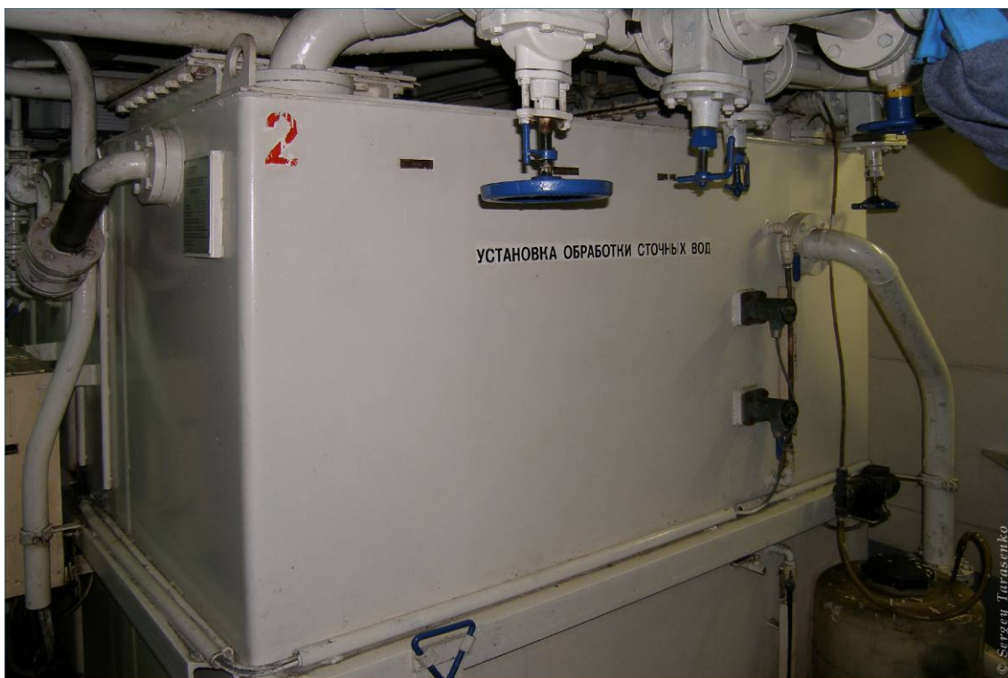
Figure 2 – UNEX BIO sewage treatment plant (Rauma-Repola, Finland) installed onboard r/v “Akademik Fedorov”
