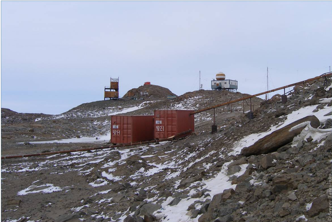
Figure 5 – Wastewater treatment plants at Novolazarevskaya station (2008)
