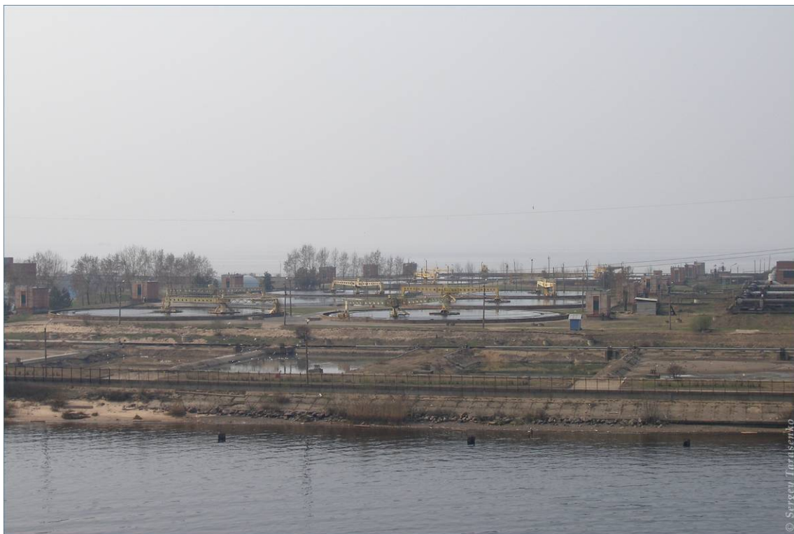
Figure 1 – Sedimentation tanks (St. Petersburg, 2006)
