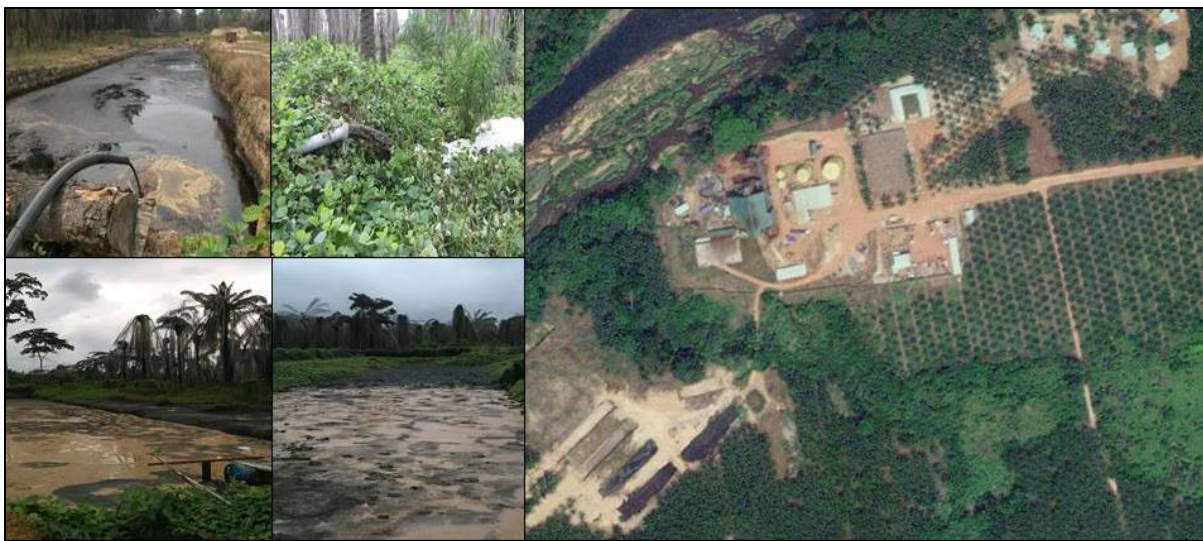
Figure 5: Goldtree pond system. The picture on the left hand corner is a bird-eye view showing 3 of the 5 ponds in use. It also shows that there is no connection to a final discharge, which is actually performed by an external pump discharging into the plantation, as shown in the top right corner. The inlet to the ponds is also a temporary installation, as shown in the top further right. The bottom right show signs of acidification and overloading.
