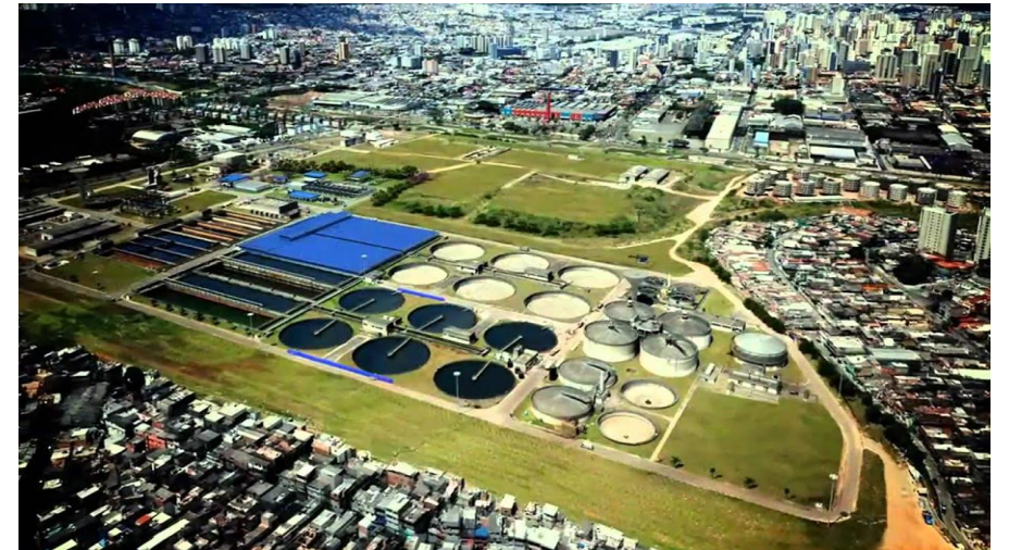
Aquapolo – Water Reuse System in São Paulo
