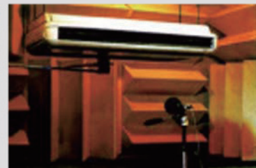
Sound test room of McQuay Shenzhen Factory, China
