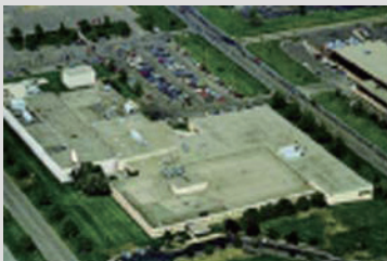
Global headquarters of McQuay (Minneapolis, USA)
