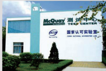
Test center of McQuay Shenzhen Factory, China
