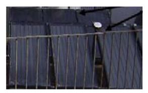
Figure 18. Flat plate solar collector array used in the desalination system [12].
