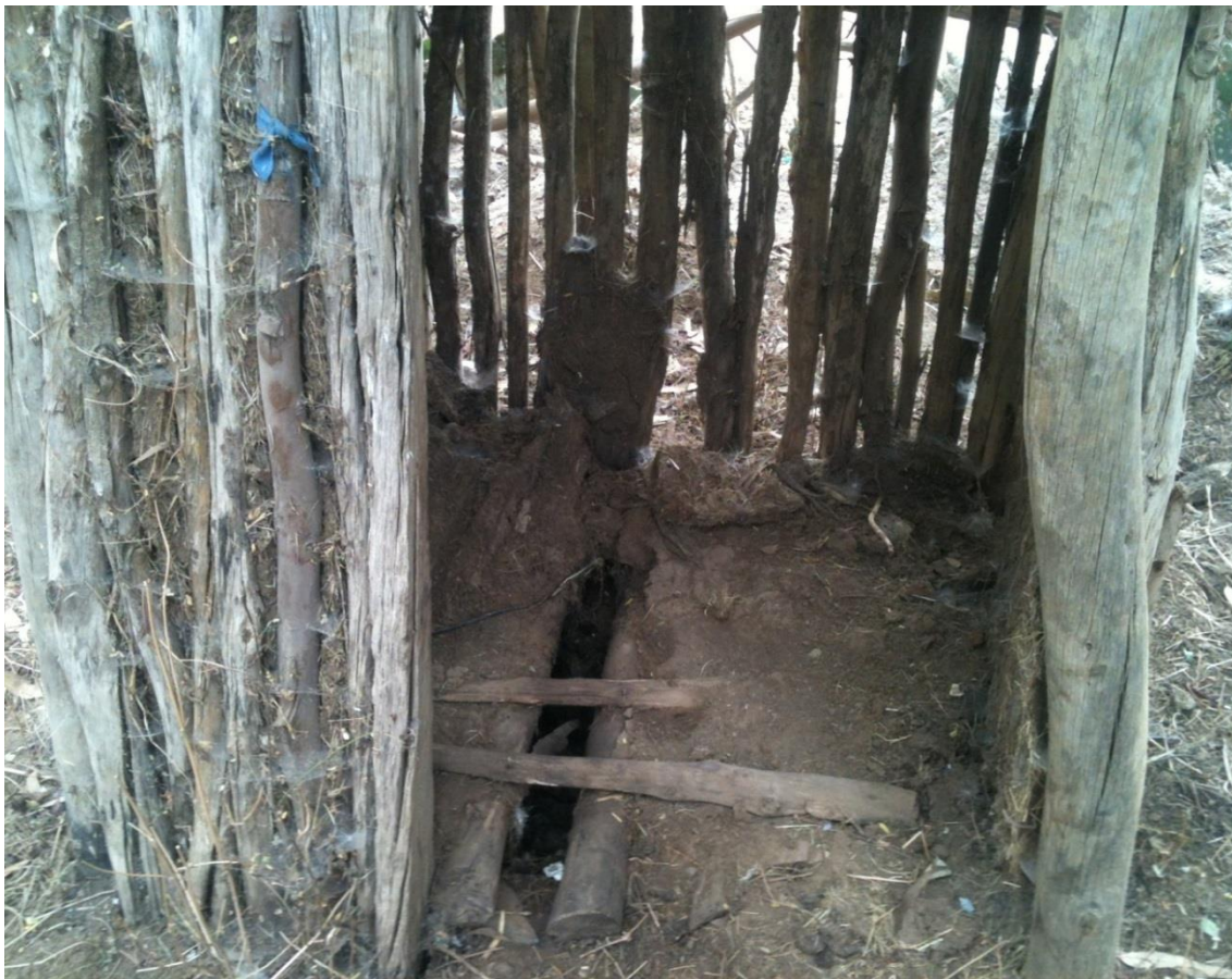
Photo: A latrine in Lumame, Amhara. "The latrine is made from sticks. There is no door. It is very open. There is no plastic covering the outside of the latrine for privacy and old feces fill up the latrine pit. However, there is no smell because it looks like latrine hasn't been used for defecating in a long time." ~Research team's notes.
