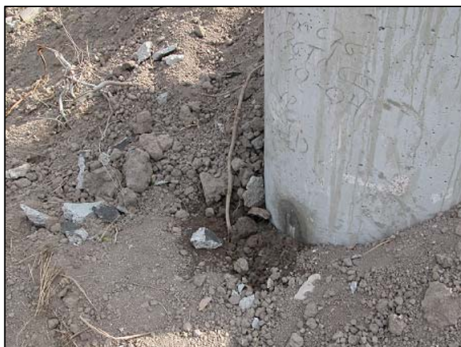
Figure 11. This photograph shows a standpipe connecting off of Lateral A-8 leaking during test. Leaks like this are very difficult to measure and are usually hard to notice.
