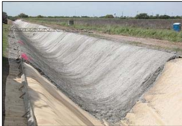
Figure 1. Layering of the new lining on Lateral A.
