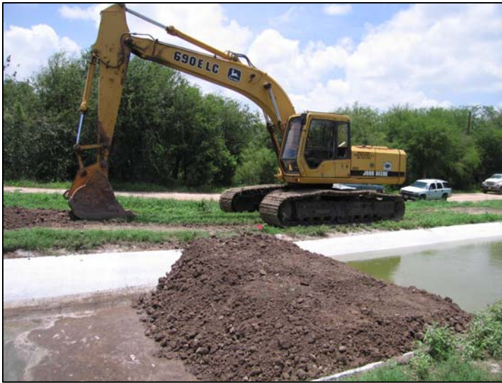
Figure 2. Backhoe used to construct the earthen dam on nonding test.
