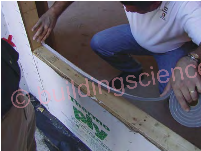
Figure 31: Weather seal gasket used as a backdam
