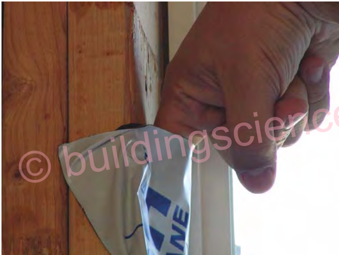
Figure 29: "Fishmouthing" of the membrane
