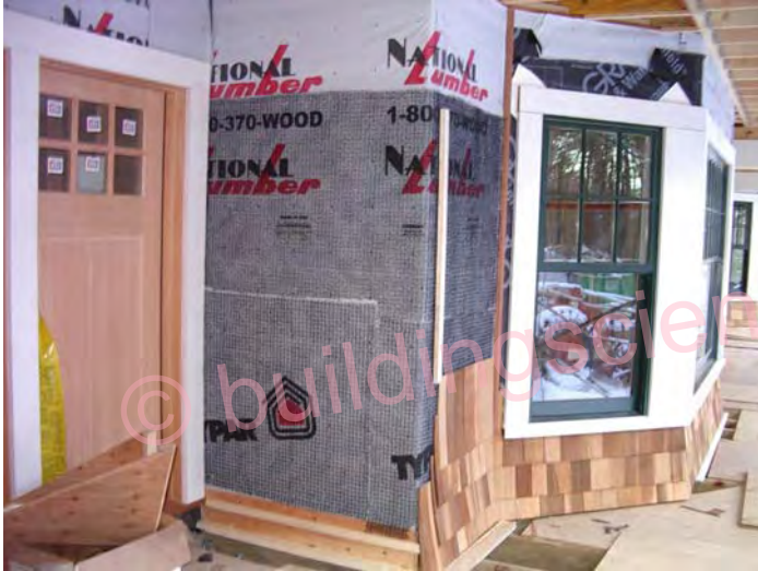
Figure 5: Drainage matt installed behind wood shingles
