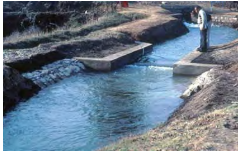
Figure 5. — A Rectangular-Throated Flume in India.
