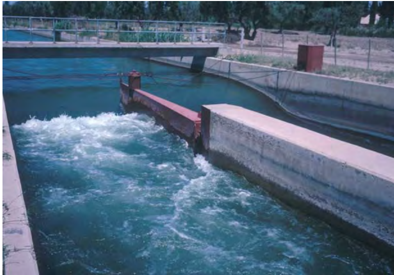
Figure 12. — Flow Division Structure with a Movable Divisor.
