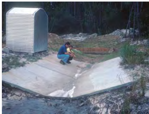
Figure 6. — Triangular-Throated Flume in Florida.
