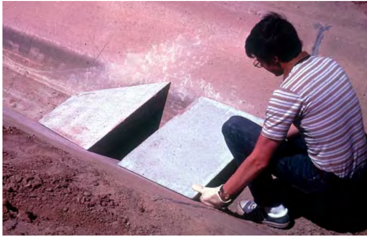
Figure 3. — Placing Pre-Cast Weir Sections in a Lined Trapezoidal Canal.
