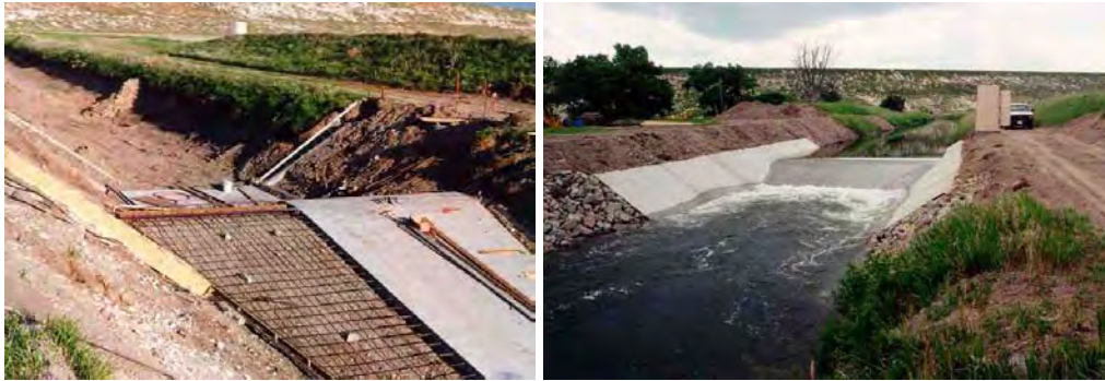
Figure 4. — Construction of a Large Broad-Crested Weir in an Earthen Channel.
