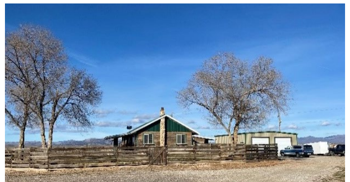
House and shop building on 15 acres in Chester, Utah.
