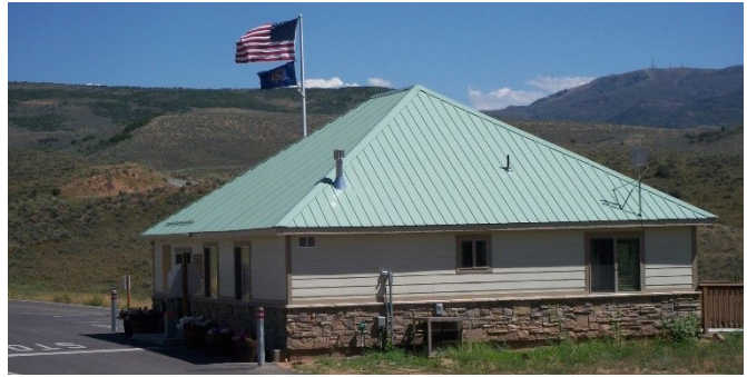
New Fee Station and Office at Entrance to East Canyon State Park. Part of the entrance realignment.
